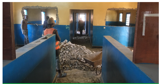
▲ Building work to open up the Surgical Ward environment
